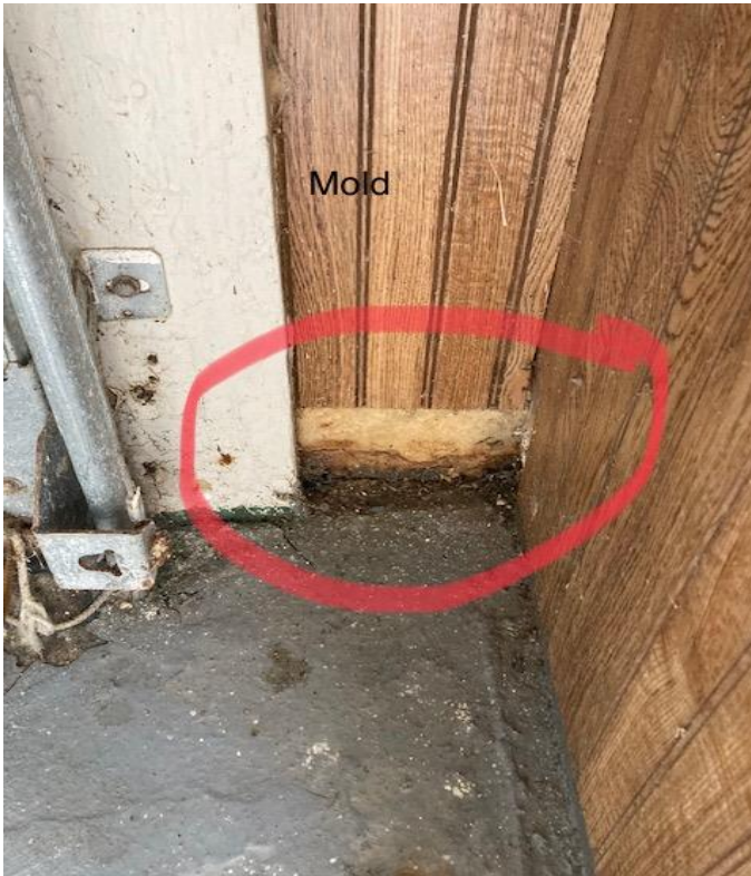
East Entrance Door by Patio
