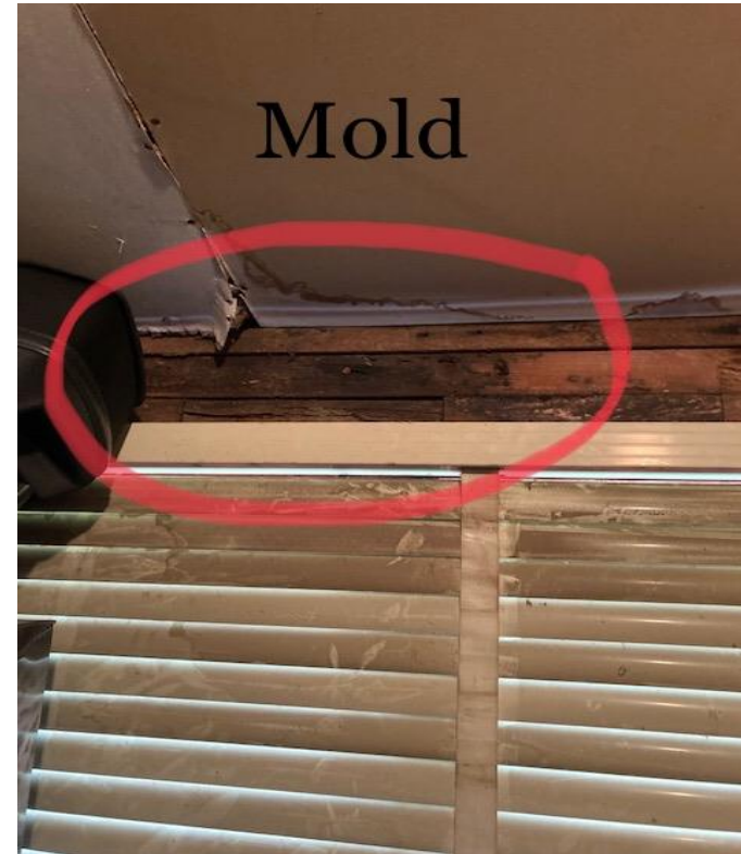
West Side Window Rob's Shop
